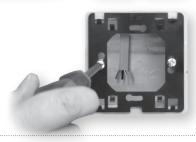
**4**: After connecting the receiver as per wiring diagram (see diagram)\*, mount the thermostat on to the backing plate and push down wire retaining clip, remount the frame.
