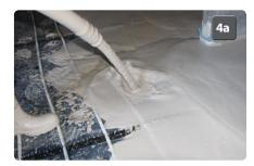
The screed should be allowed to dry naturally and under no circumstances should the underfloor heating system be used to speed up the drying times as this could effect the integrity of the floor. Once the screed has fully dried, heat from the underfloor heating system can be introduced slowly, by raising the flow temperature gradually over a period of a week until the desired temperature is reached (max 45° C).
