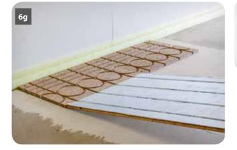
Once the first strip of end/transitional panels have been laid, apply more adhesive in a strip approximately 1250mm wide, parallel to the wall **(6g)**, again leave adhesive to become tacky and commence laying main panels, working towards the opposite wall.
