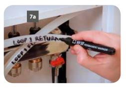
Always begin laying pipe at the manifold allowing a bit extra for final connection to the manifold identify each loop flow, return and loop number using a permanent marker (7a).
