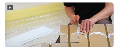
wundatherm 'Acoustic' Boards are designed for easy installation, cutting to shape where required. Transitional pipe runs, additional corners, bends and extra pipe channels will normally be required and are simply cut from a panel using a hand saw, electric jigsaw or a router to cut additional channels (5c, 5d).
