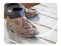
Walk the pipe into the channels in the overfloor boards ensuring the pipe is pushed securely into the bottom of each channel (7b).
