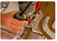
Using a router with bit set to 17mm depth gentle cut the new channel following the marker pen layout **(H)**. Ensure the channel is clear and free from debris, if required the channel can be lined with aluminium tape. Lining with aluminium tape is not required in areas with highly concentrated/close floor heating pipes.
