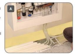
Recess mounted cabinets are designed to be fitted into a wall or opening before installing the floor heating system and pipes.
