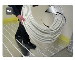
This will help deter the pipe from trying to twist and keep tension pointing downwards, ease the pipe around and into the bend. Lay the pipe into the return or corner, gently forming and pushing the pipe into the channel as it works around the bend **(9d/e)**.
