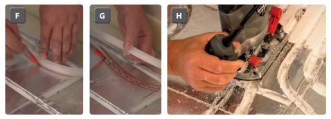
Using a router with bit set to 16/12mm depth depending on pipe, gently cut the new channel following the marker pen layout **(H)**. Ensure the channel is clear and free from debris, if required the channel can be lined with aluminium tape. Lining with aluminium tape is not required in areas with highly concentrated/close floor heating pipe .
