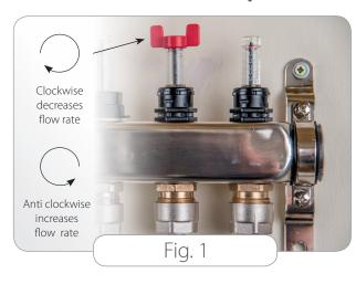
IMPORTANT: Adjust flow rate by hand only using the supplied red adjustment key. Do not force the flow gauge beyond fully open, as this will cause damage to the flow meter. Do not use pliers or grips to adjust or over tighten the flow gauges.
