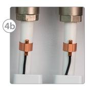
Auto balancing actuators must be wired in accordance with Wunda wiring guide. When the floor heating system is fully commissioned and thermostats call for heat, each individual actuator will activate and self-calibrate.
