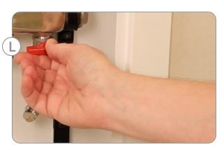
If pressure drops investigate and remedy, the mains water supply hose can be removed, leave the drain hose in place as this will be required to release the pressure at a later stage. It is good practice to leave the system under pressure whilst laying of final floor finish to indicate any possible damage to the loops of pipe.
