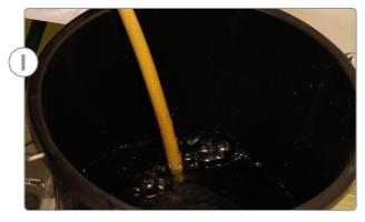
When a steady flow is achieved and ALL air has been passed, close the manual return valve on the return bar, leaving the flow gauge open. (pic G previous page) Repeat this exercise with each individual loop, one at a time.
