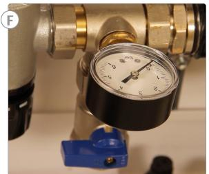
Connect the mains supply hose to the top flow red tap. Connect the drain off hose to the lower return blue tap, place the end of the drain hose into a bucket. Open both the red and blue drain taps, turn on the mains water supply to the fill hose.
