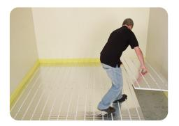
(Take care when cutting the boards, wear work gloves as the aluminium can be sharp. Keep any offcuts as these may be useful in other areas. If you cut boards incorrectly don't worry, you can bond the 2 halves in a main panel area.)
