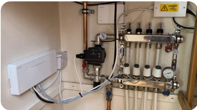
Remove all of the manual return valve caps and fit the electronic actuators in their place. Keep the manual caps for future use as they are useful if ever re-filling or purging the loops of air.
